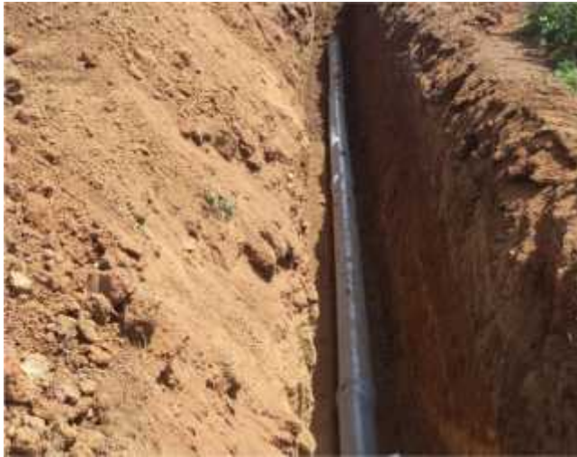
LAYING OF DN 200 uPVC
