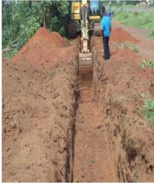
EXCAVATION AND LAYING OF DN 350 LARGE DIAMETER STEEL PIPE
