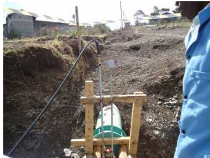
PRESSURE TESTING OF DN 350 PIPELINE
