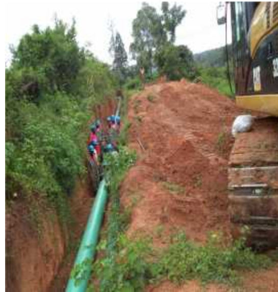
EXCAVATION AND LAYING OF DN 350 LARGE DIAMETER STEEL PIPE
