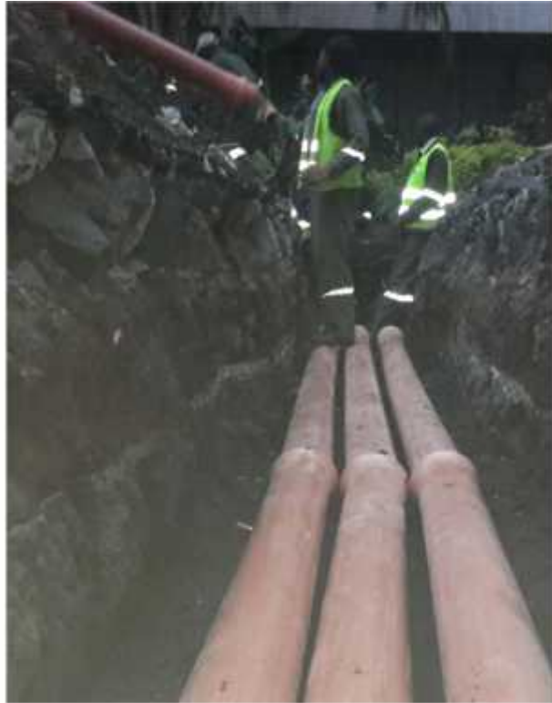
EXCAVATION AND LAYING OF UNDERGROUND HIGH VOLTAGE POWER CABLES
