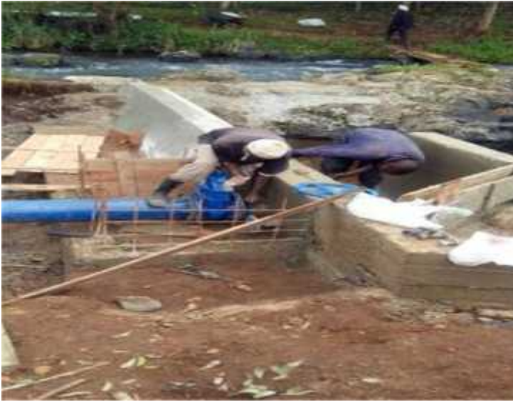
CONSTRUCTION OF WEIR AND INTAKE WORKS
